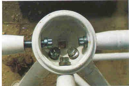
Fig.22 SPHEROBAT system node
