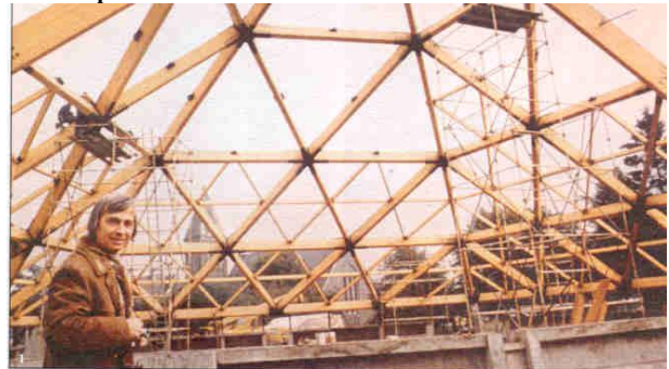
Fig.17 Wooden structure of the church in Libramont
