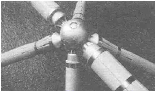
Fig.20 Node of structure with bamboo members
