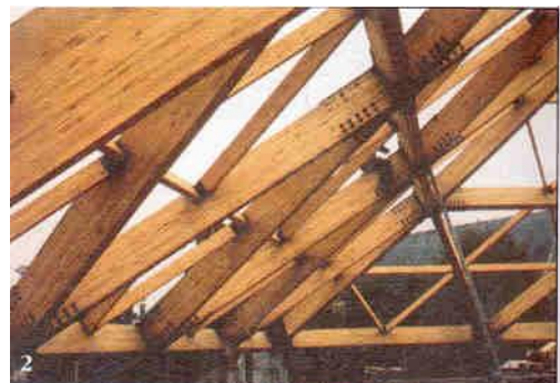
Fig.18 Closing up of wooden structure of the church in Libramont
